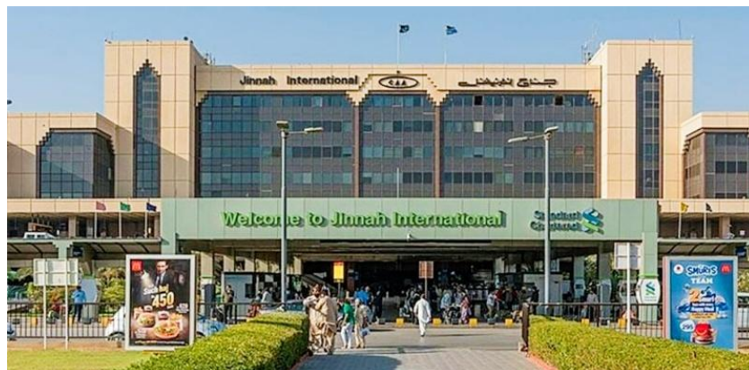
Figure 1. Front View of Jinnah International Airport, Karachi.
